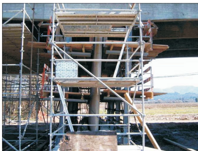
Fig. 4. Example of scaffolding system used to access the test site
