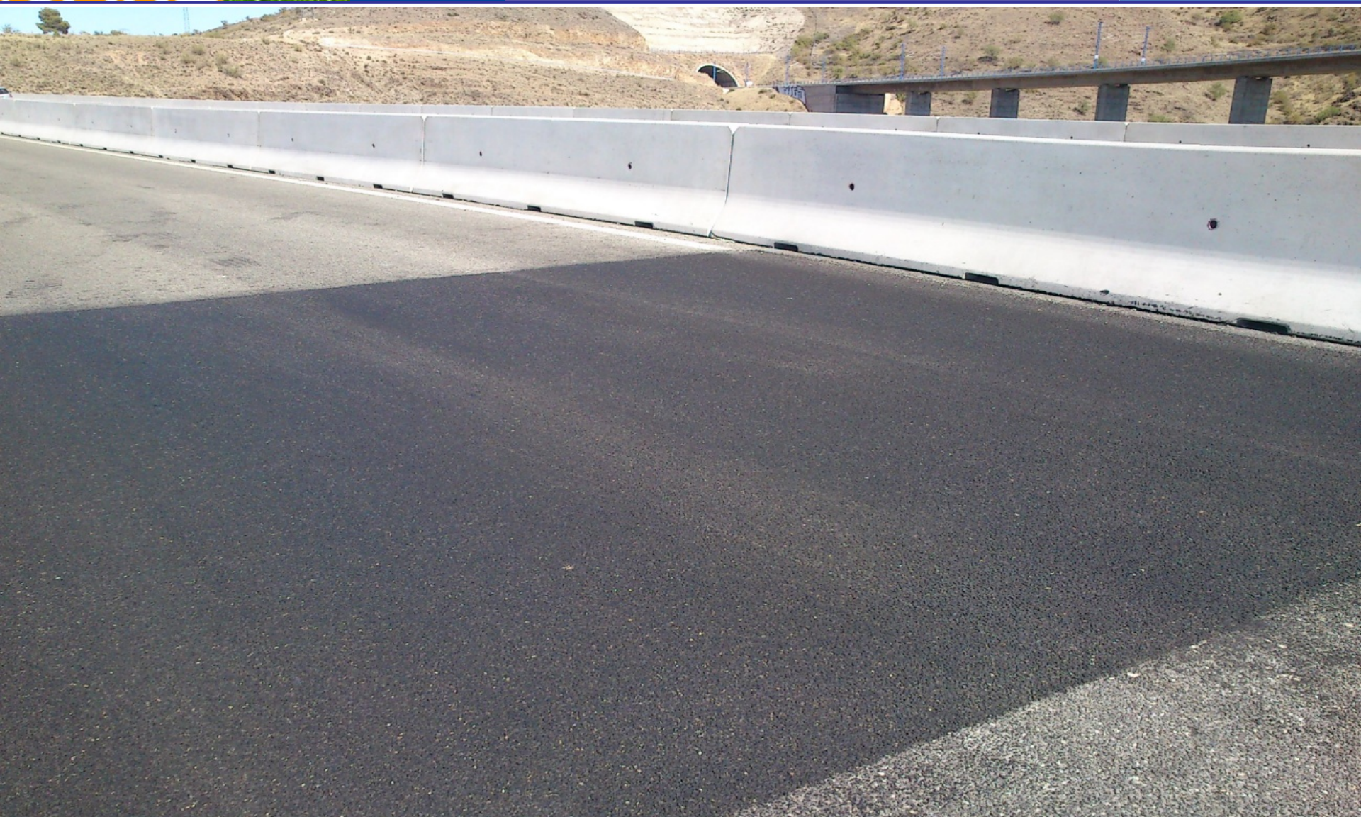
Invisible expansion joints in existing bridges
