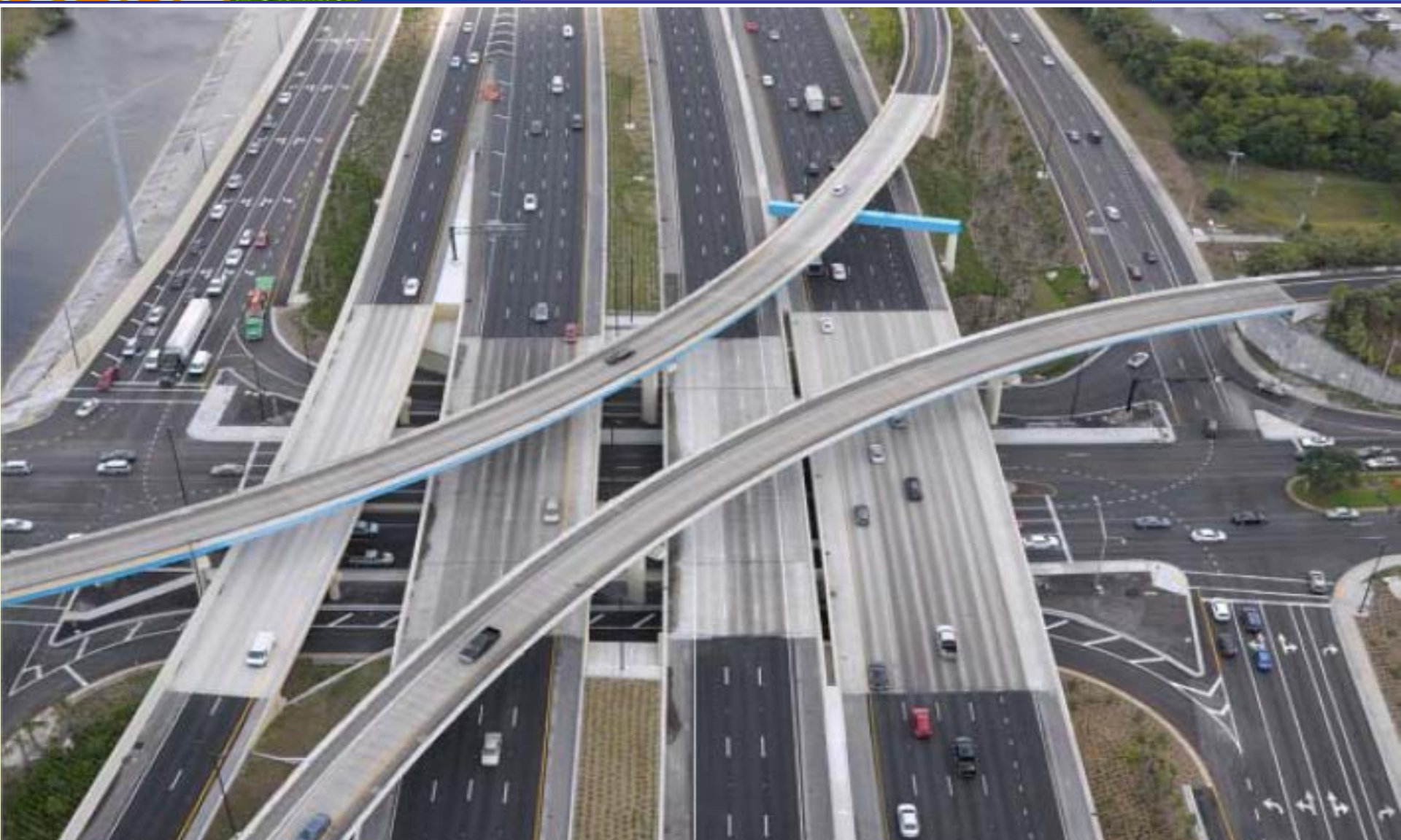
Change geometry - Jacking of existing access ramp to a new position
