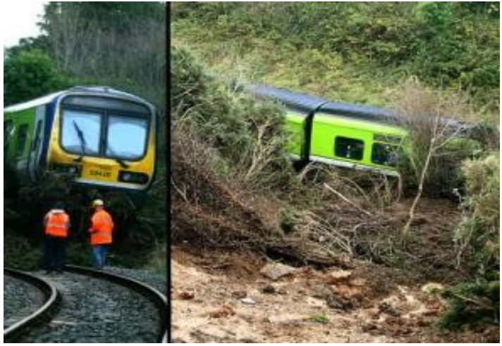
Rainfall induced slope failure outside Wicklow station (2009)
