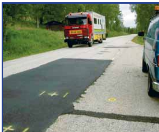
Truck traversing strain gauge
