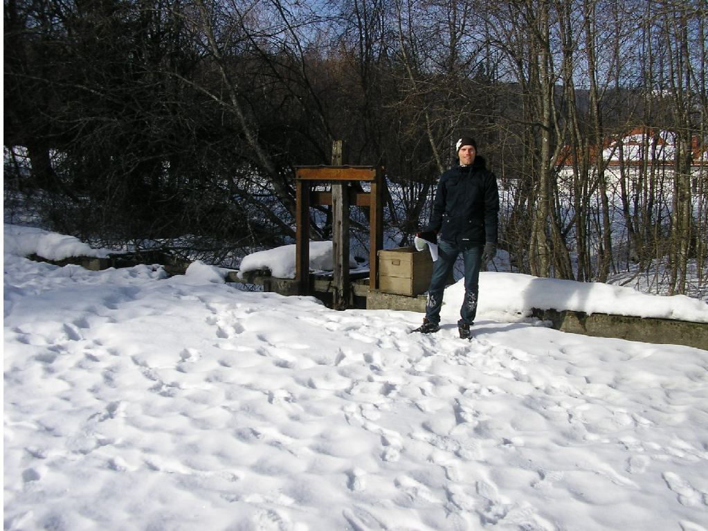
Figure 2: Old timber floating dam critical to collapse (Photo, SGI).
